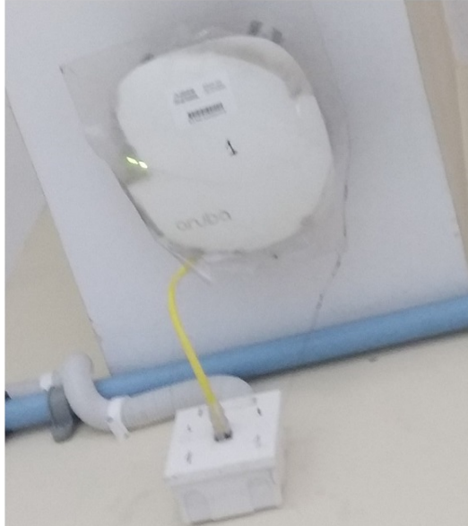
Figure 8: Physical placement of a certain AP on the ceiling of experimental area.
