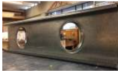
(b) Section with edge-stiffened holes
